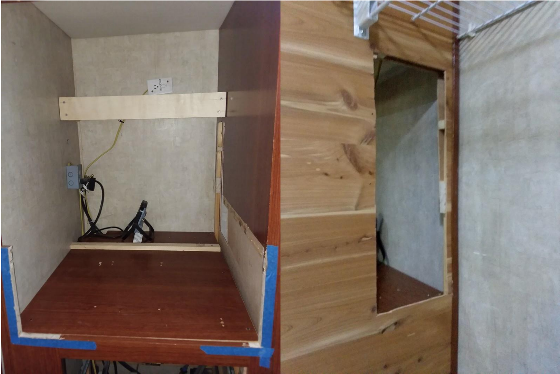
Jim and I easily picked the dryer up and put in place. I needed to perfectly locate where the hole for the dryer vent needs to be. I'll admit to being a bit nervous about drilling a 4" hole in my beautiful coach!!!!
