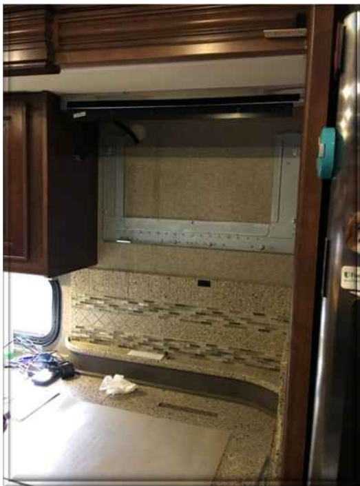
One more lift to get it in the vacant space
