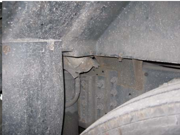
Broken bracket aft of right rear tire
